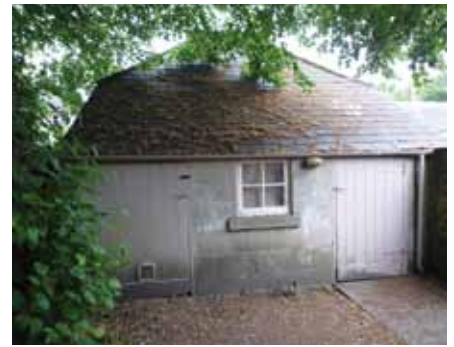
Combe Hay Manor Gas House
