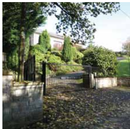
Inappropriate boundary treatment that is discordant with the character of the Conservation Area
